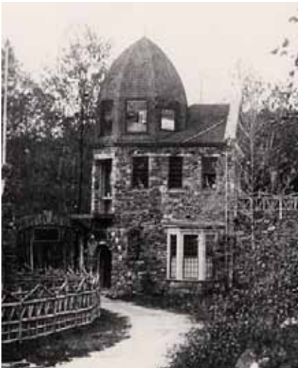
The Caretaker's Cottage once had two stories.
