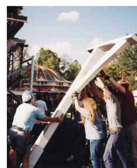
Volunteers raise the last column of the Bumper Car Pavilion.
