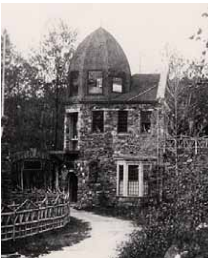
The Caretaker's Cottage once had two stories.
