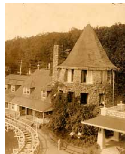
The stone tower in the 1920s
